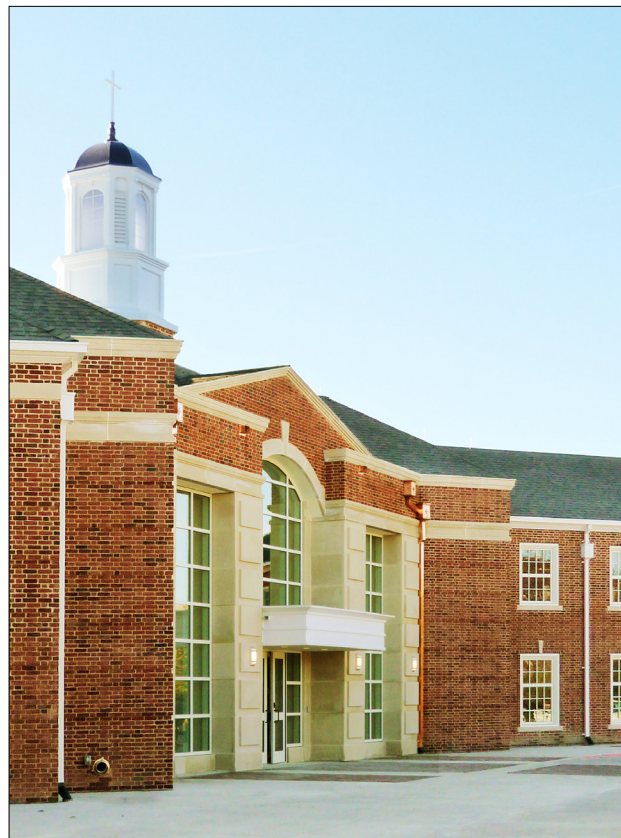
The new entrance was designed to stay true to the traditional style of architecture.
